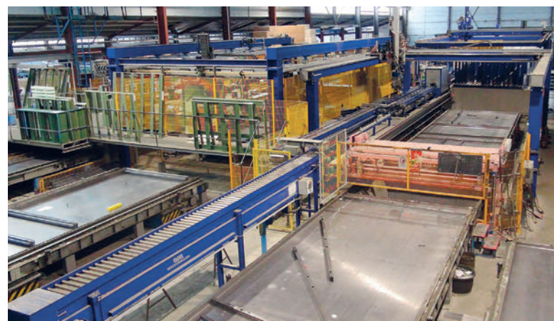
Fig. 2: Overview of the magnet box handling system, shuttering/stripping robot (at one position), with pallet and shuttering cleaning unit, storage robot and robot for placing inserted components
