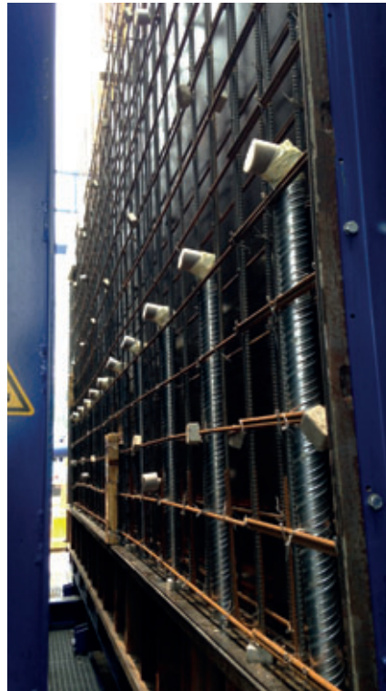
View inside a cavity prepared for concreting
