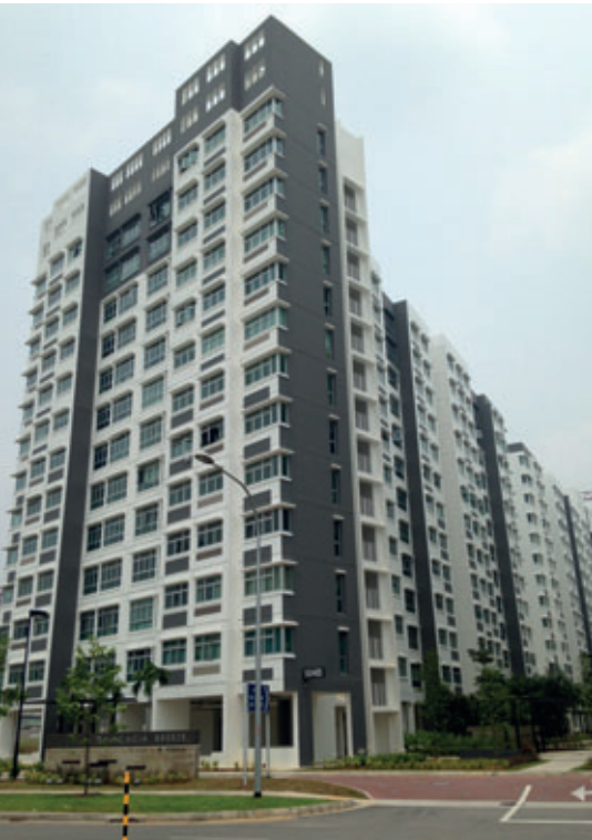
Residential complex built from precast elements
