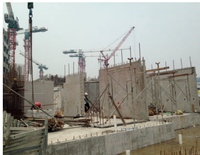
Installed precast concrete walls
